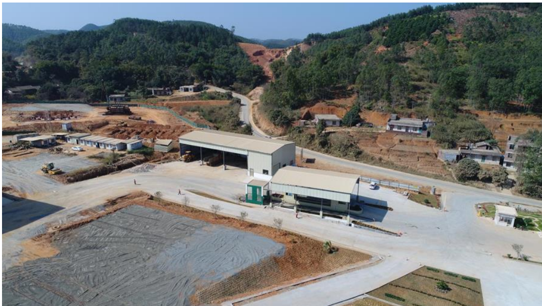
Cenxi Haoyi Construction Waste Material Recycling Facility
