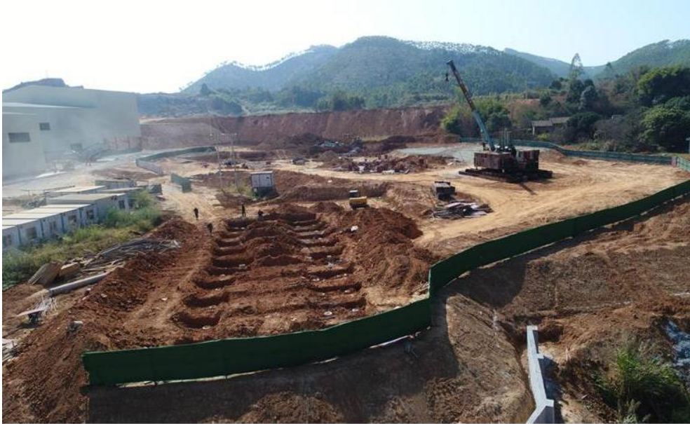
Construction of Cenxi Xing Jian in progress.
